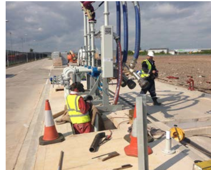
Installation of 3 arm bottom loading skid
