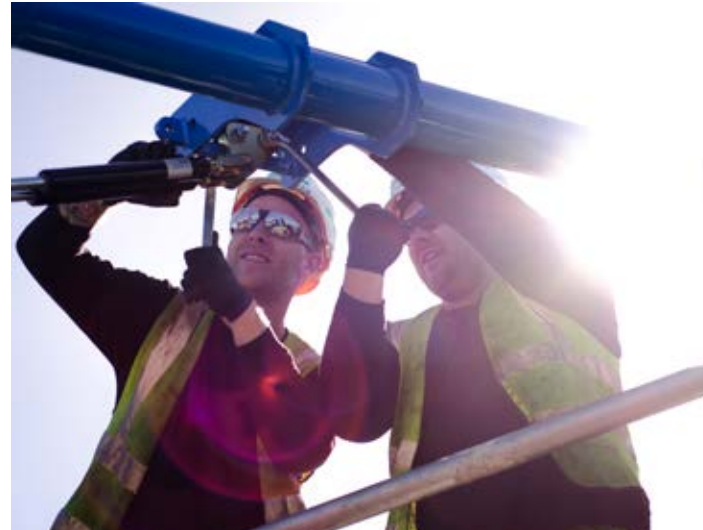
Balance adjustment for loading arm
