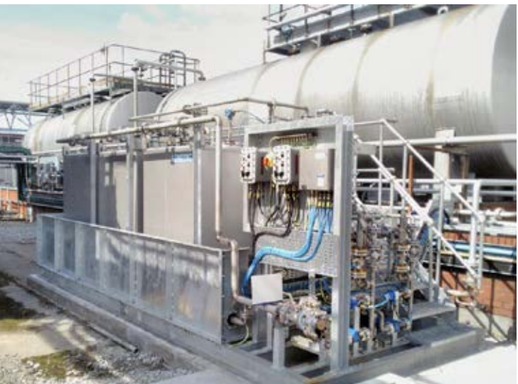
Additive Injection skid with duty and standby metering - UK - Fuels Industry
