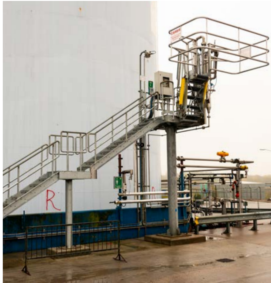
Fixed Access Platform with 5 step folding stair and top loading arm - UK - Chemical Industry
