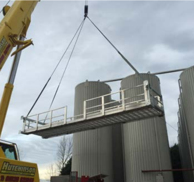
Installation of VLP Cage section
