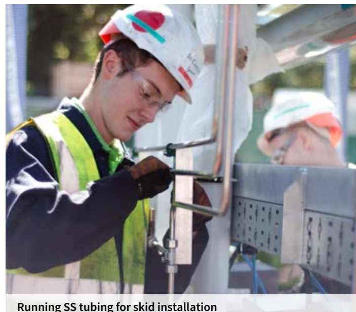
Running SS tubing for skid installation
