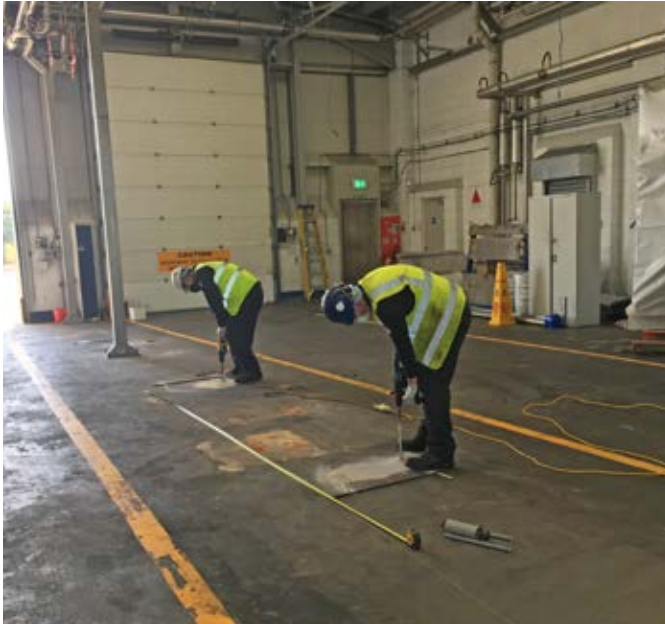
Drilling Floor ready for platform column install
