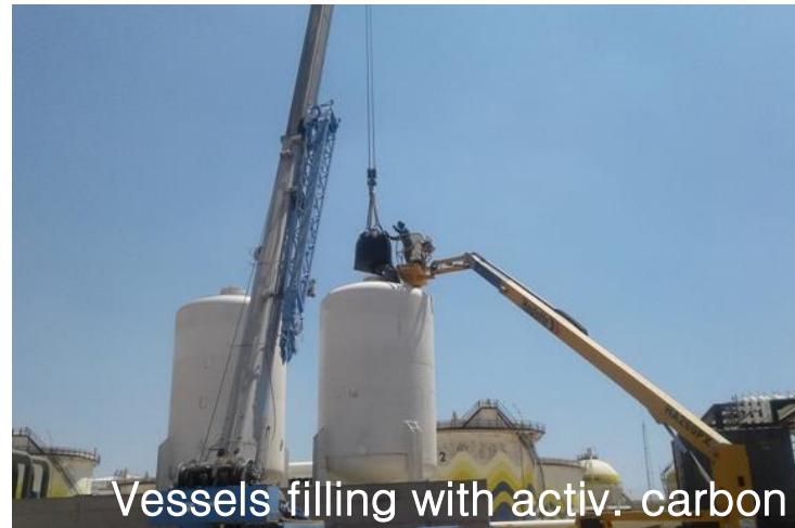
Vessels filling with activ. carbon
